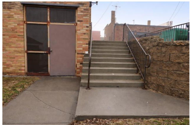
5 North Entrance to Upper-Level Former Library
