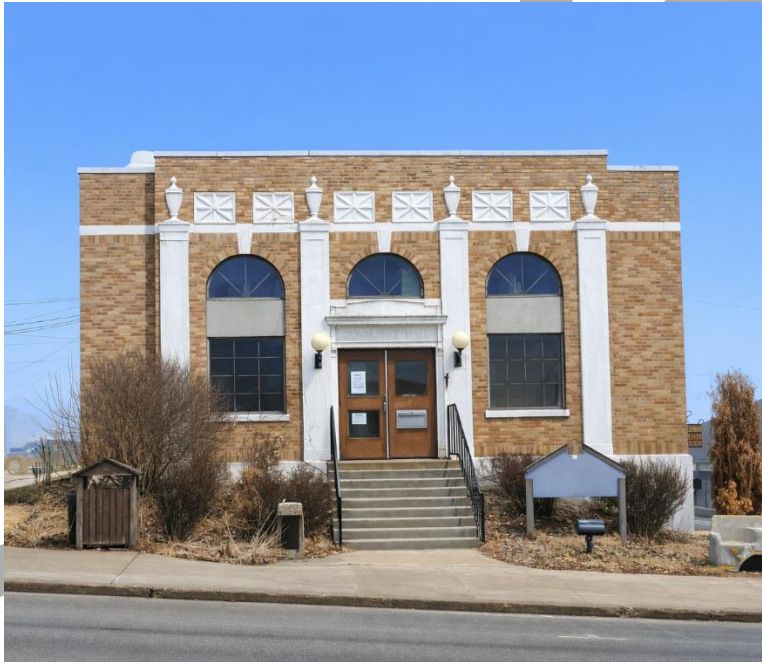
1 Ellsworth Former Library Building, Main Entrance to Upper Level, Pictured Above
